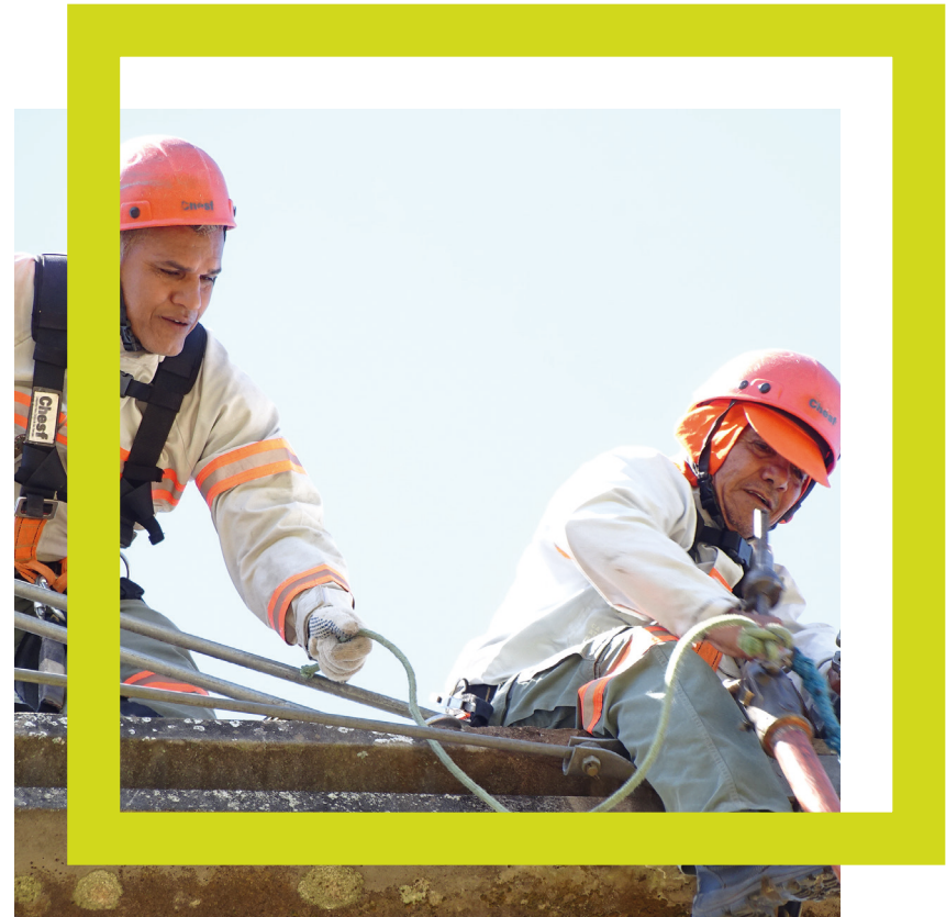
Chesf professionals perform maintenance work on transmission lines
